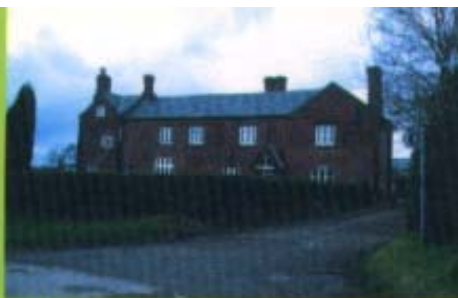
South Facade- Girt Woolden Hall
